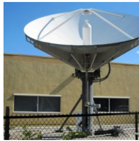
Vertex 6.3M KPK Cassegrain KU-Band Antenna
