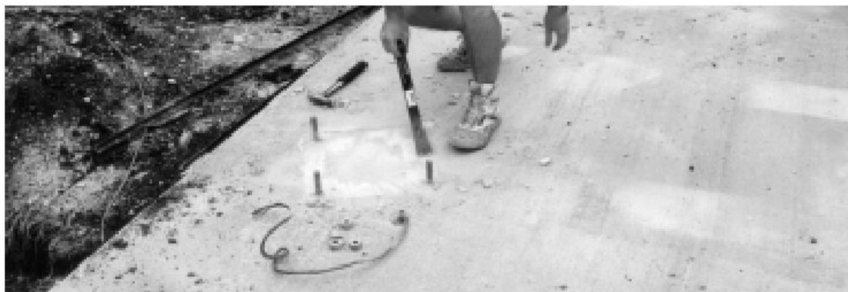
FIGURE 1-2: SCRAPING FOUNDATION PADS
