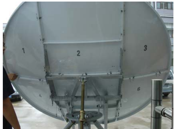
put the reflector on the bracket of the antenna
