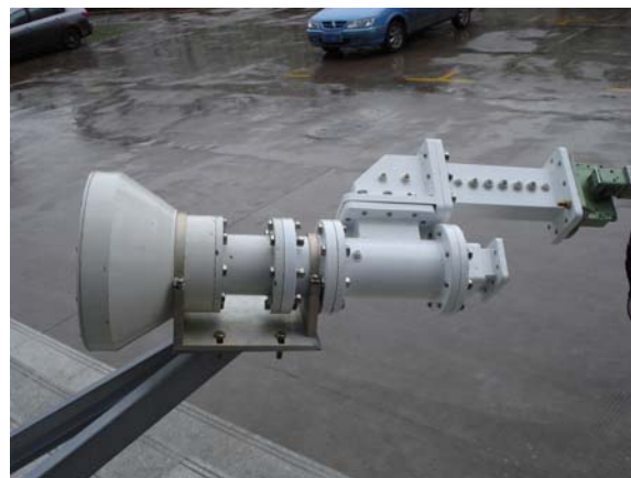
the installation of the feed and the coaxial duplexer
