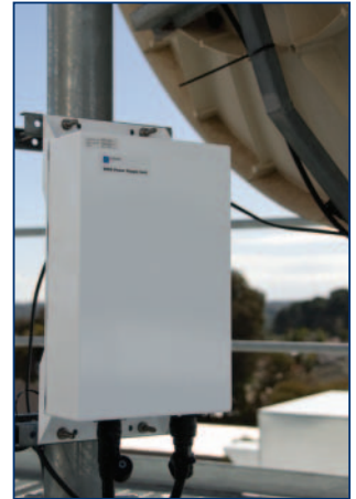
6582 Transformer Power Supply Unit
