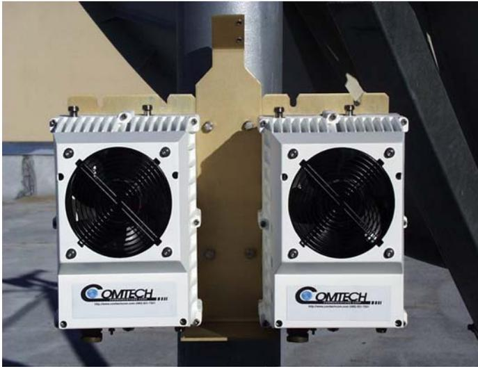
**Figure A-19. Installation of XSAT Transceivers**
