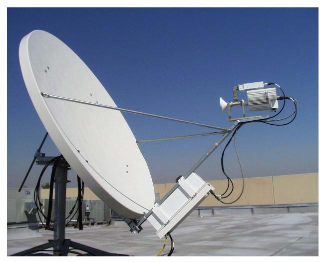
Figure C-1. KST-2000A Single Thread System Installed on Spar Arm.
