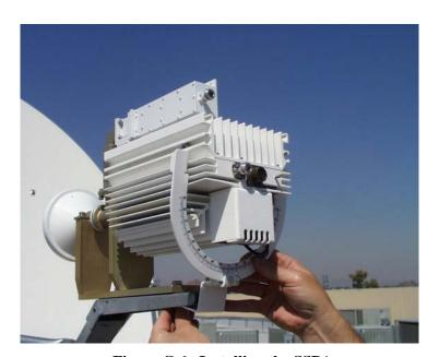
Figure C-6. Installing the SSPA
