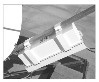
Figure C-2. Typical Converter Unit Installation on Spar
