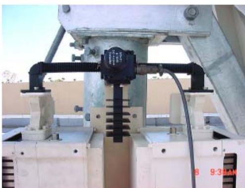
Figure C-19. Installation of the Waveguide Switch.
