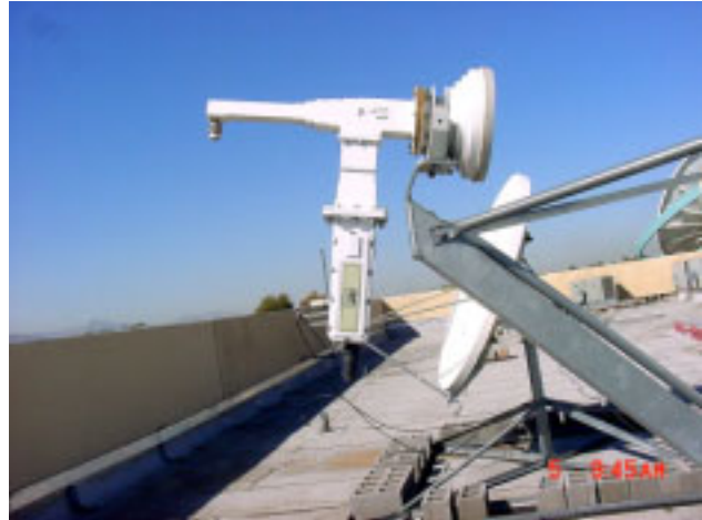
Figure 2-8. Installation of LNA
