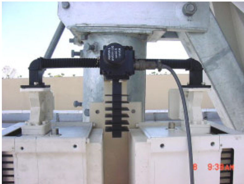
Figure 2-25. Installation of the Waveguide Switch.
