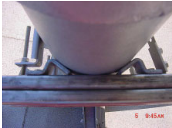
Figure 2-24. Looking down at Pipe Blocks
