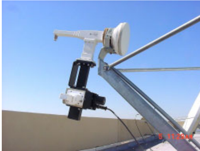
Figure 2-26. Installation of the Redundant LNA Assembly.
