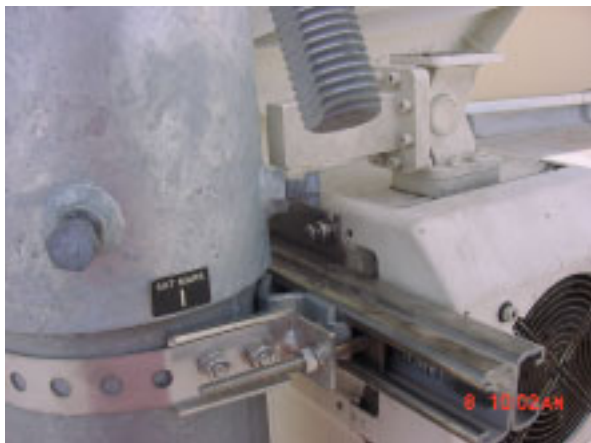
Figure 2-5a. Installing the Pole Bracket
